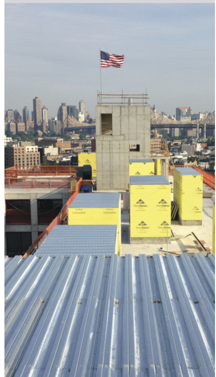
PHOTOS: SKYLINE RESTORATION INC.
